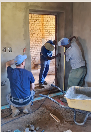
Installation of electricity
