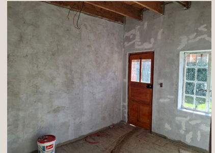
Plastering and new door
