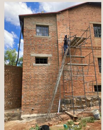
Reconstruction of two walls
