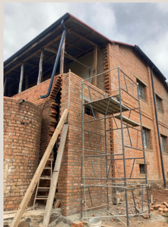
Reconstruction of two walls
