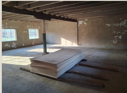
Plastering and new cement floor
