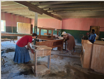
Clearing of room
